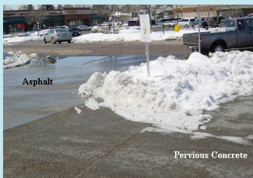
Pervious pavement & snow ( www.perviouspavement.org )
