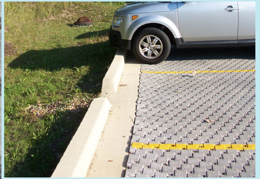
A parking lot of pervious pavement (Megan Riechmann)
